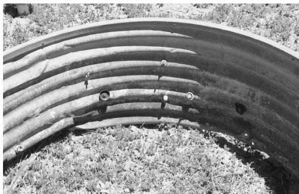
**Figure 24 – Prior Repairs to Drinker**
