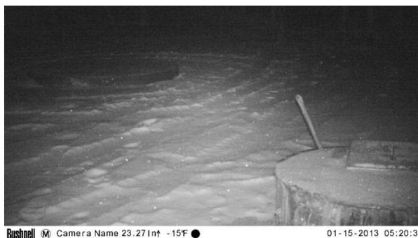
**Figure 29 – Ice Covered Float Tank at - 15 °F**
