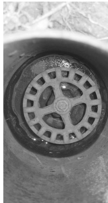
**Figure 27 - Water in Valve Box**
