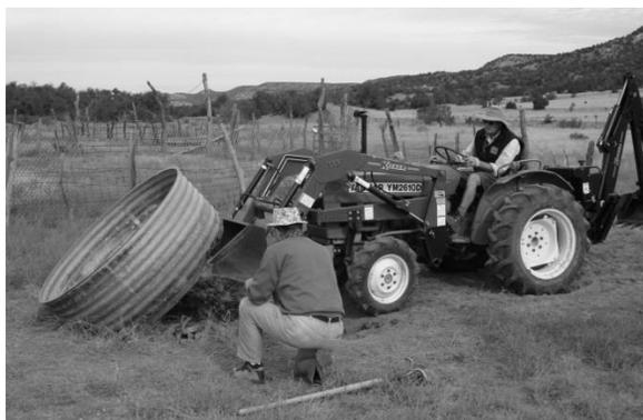
**Figure 23 – Removal of Leaking Drinker**
