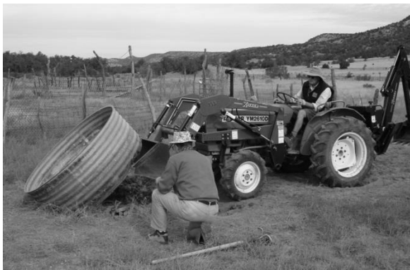
Figure 23 – Removal of Leaking Drinker
