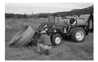
Figure 23 – Removal of Leaking Drinker
